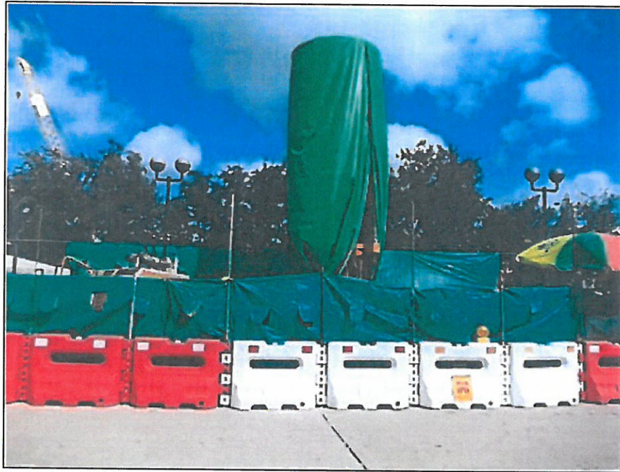
Photo 3 – Enclosure for Drilling Plant
