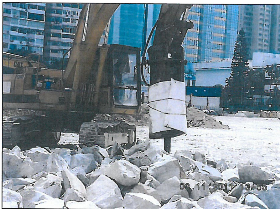
Photo 4 – Breaker Tips were wrapped with noise absorbing material
